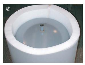
Pictures showing how to mount soft-foam insulation with a PVC sheet on a storage tank.
