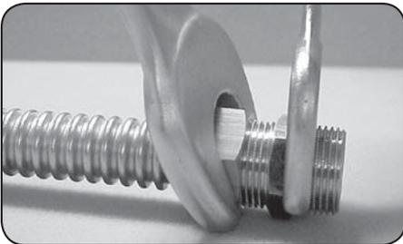
Tighten the double nipple to close up the existing trough to an evenly sealed position.
