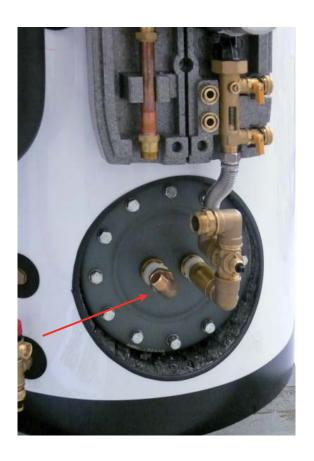
8. Fit the T-piece (code 7180) to the elbow and the reducing hex nipple (code 7697) to the T-piece, see fig. 9.
