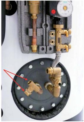
9. Fit the pipe (code 3012) to the T-piece. Then turn the assembly to a vertical position and attach the pipe to the Solar Pump Station, see fig. Fit actuator onto the zone valve.
