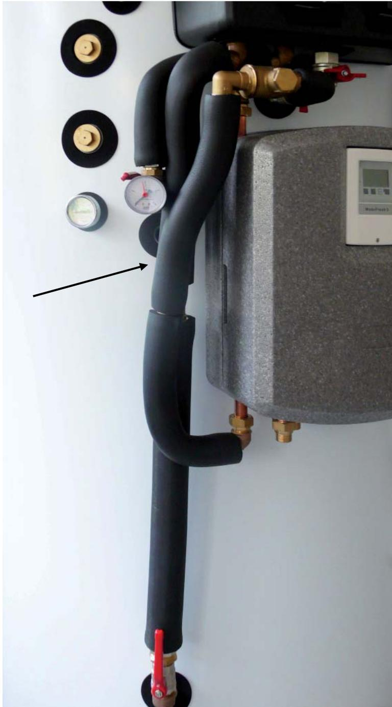
2. Remove the 3/4" pipe connecting the freshwater station with the T-piece assy.
