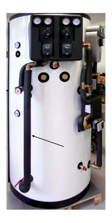
2. First remove the 5/4"x1" reducing hex nipple from the pump station and then remove the 1" elbow FM.
