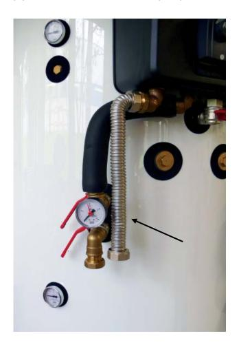
8. Fit the zone valve assy (code 13156) as shown in the fig.
