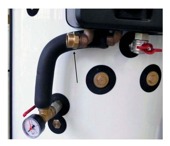
4. Remove the 5/4"x1" reducing hex nipple from the lower connection point and fit it to the already removed 1" FM elbow. Fit this newly created assembly to the valve as shown in the fig.
