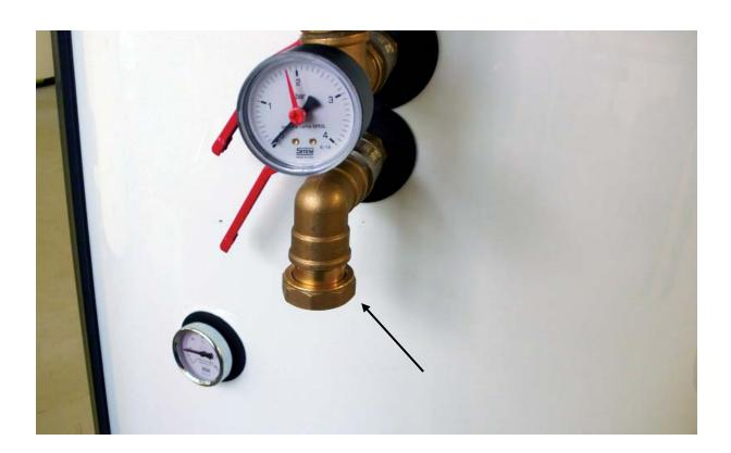
7. Cut insulation to circa 500 mm and slide it onto the 5/4" pipe, 390 mm long (code 13965). Then fit the complete pipe to the outer elbow of the pump station.
