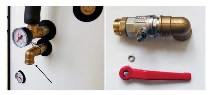
6. Fit the fitting (code 12217) to the ball valve assy.
