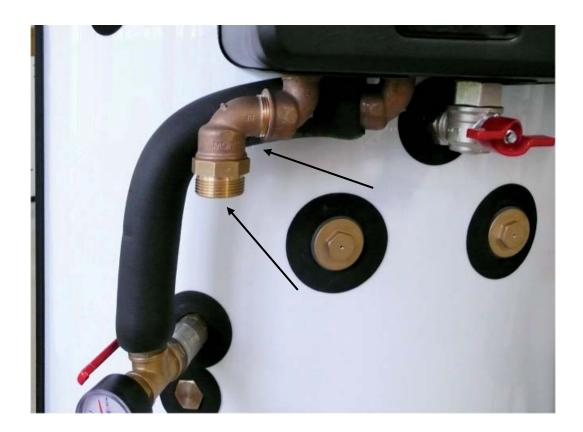
3. Fit the 5/4"x1" reducing hex nipple from the previous point into the elbow on the pump station.
