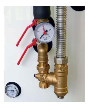
9. Cut insulation to circa 700 mm and slide it onto the 5/4" pipe, 670 mm long (code 13966). Using this pipe, connect the zone valve with the ball valve assy. Fit the actuator onto the zone valve.
