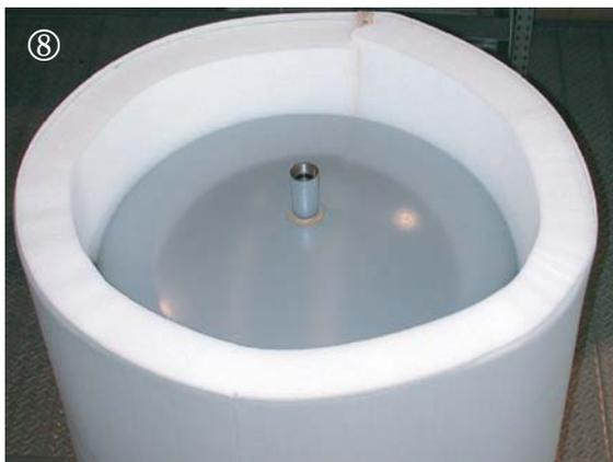
Pictures showing how to mount soft-foam insulation with a PVC sheet on a storage tank.
