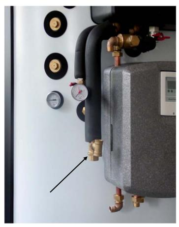
5. Remove the plug below the pressure gauge assy and fit the zone valve connection assy (code 13967) in its place. Remove the handle from the assembly prior to fitting and then return it back.
