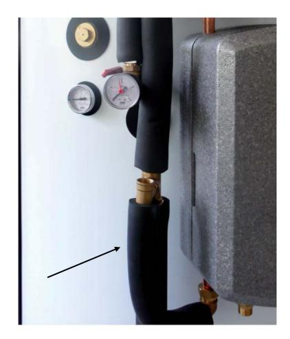
3. Remove the 5/4" pipe connecting the elbow assy with the T-piece assy.
