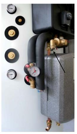
7. Slide insulation onto pipes codes 3012, 13997 and 13999, then fit the pipes to the zone valve assy (code 12688). Remove the actuator from the zone valve and the fittings from the zone valve's B port.
