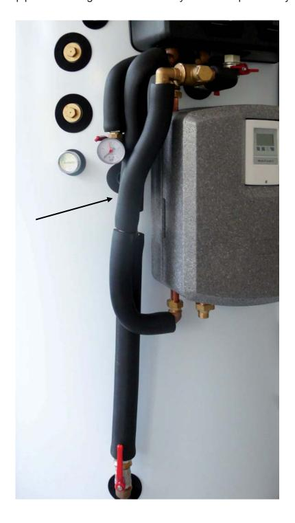
2. Remove the 3/4" pipe connecting the freshwater station with the T-piece assy.
