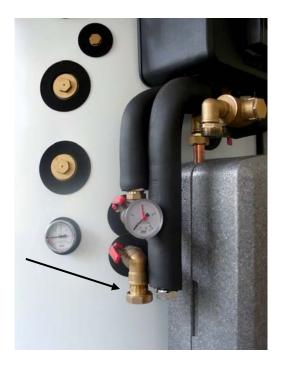
9. Fit the zone valve assy and interconnect it as shown in fig. Fit the actuator onto the zone valve.
