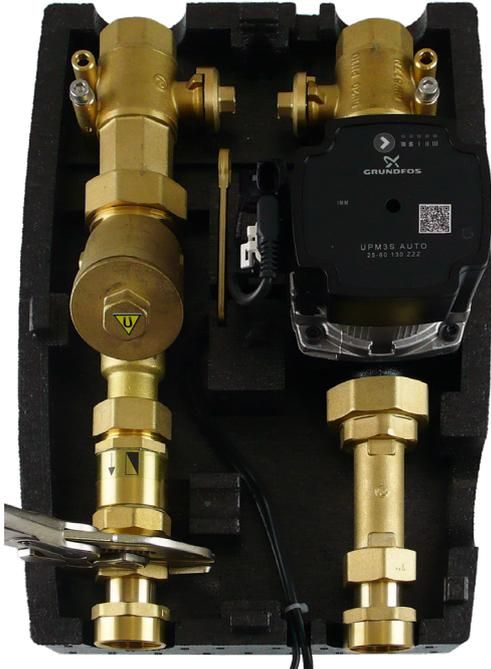
Install the union 15695 in their place, then attach the ball valve w. drain valve (17415) to the union.
