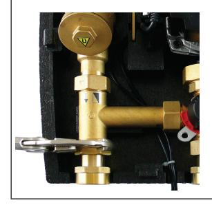
Install the union 15695 in their place, then attach the ball valve w. drain valve (17415) to the union..
