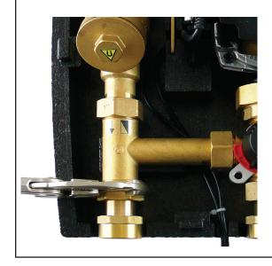
Install the union 15695 in their place, then attach the ball valve w. drain valve (17415) to the union.
