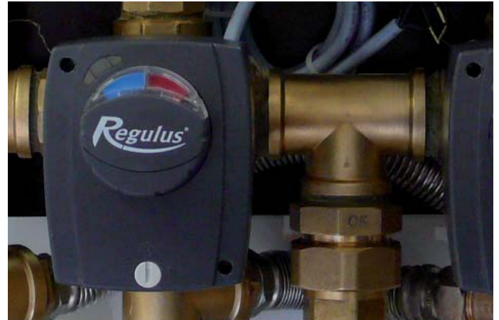
32. Mount the actuator onto the left-hand mixing valve.
