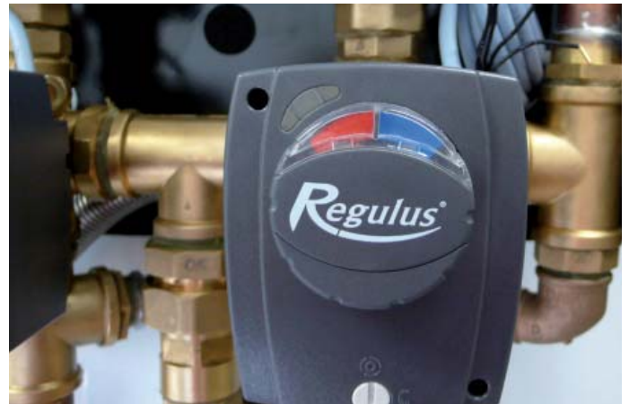
17. Mount the actuator onto the right-hand mixing valve.
