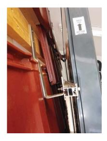
For solar collector installation onto a sloping roof, roof anchors are used that shall be fastened to rafters, or to an auxiliary board. Roof anchors shall be selected with respect to the roofing type and composition. The most popular and suitable for current roofing types are roof anchors in stainless steel or hot dip steel. For flat roofs, these are bolts with clamp for fastening H beams.
