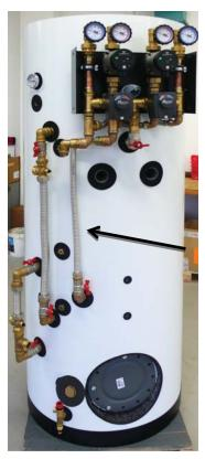
21. Locate the 1" hex nipple (in the Zone Valve Assy) fitted as shown in point 13 and the 1" Elbow Assy fitted as shown in point 9. Connect these two using the dedicated 1" pipe, 1010 mm long, code 13481. Fit the actuators to zone valves.
