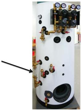
19. Locate the Zone Valve Assy fitted as shown in point 5 and the Elbow Assy fitted as shown in point 16. Connect these two using the dedicated 5/4" pipe, 490 mm long, code 13488.
