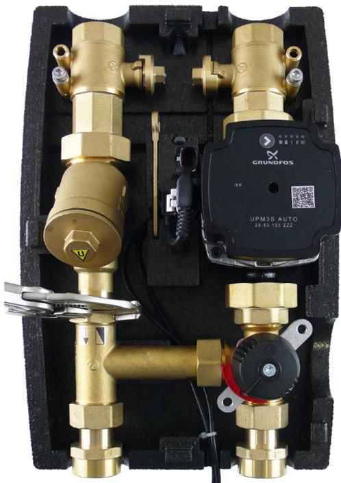
Remove the filter and install the replacement piece 19017 in its place.
