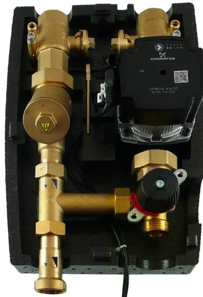
Install the extended union w. check valve, code 18797, to the flow pipe.
