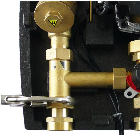
Install the unions 15695 in their place and the ball valve with drain valve 17415 onto each of them.
