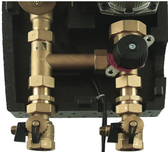
**C – Union, 1" Fu/F, extended, with check valve incl. gaskets**
