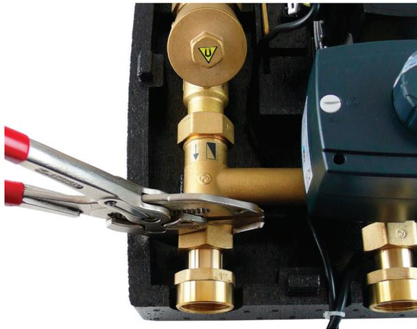
Install the union 15695 in their place, then attach the ball valve w. drain valve (17415) to the union.
