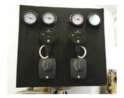
26. Fit the plastic cover onto the pump station with 4-way valves and fix it with 4 plastic screws M6x10 (code 12713).
