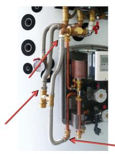
21. Using the 5/4" pipe 580 mm long, connect the T-piece assy with the ball valve assy.
