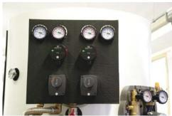
25. Connect the terminals of the pumps with cables, push the cables behind the insulation.
