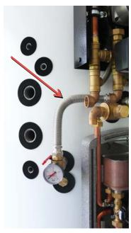
18. Fit the 1" pipe 410 mm long (code 11271), connect the zone valve assy with onto the pump station.
