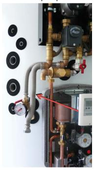
19. Fit the 3/4" pipes 320 and 450 mm long (code 3041) to the T-piece assy (code 13983). The 450 mm long pipe shall be fitted at the right-hand side, see fig.
