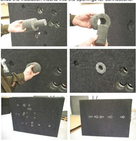
3. Fit on the front insulation part, then the rear insulation part. Check the proper position of the insulation towards the sockets prior to final fixing. Use the jig to close the locks.
