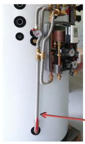
22. Fit two thermometers (code 10474), included in Kit 13237, and 6/4" and 1/2" plugs or electric heating elements and a safety thermostat.
