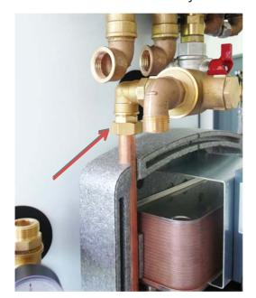
14. Fit the solar pump station (code 14866) using 2 screws M6x16 and washers (codes 12996 and 7853) - all these components are included in the Kit code 12227.
