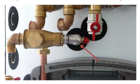
13. Connect the TSV3B assembly with the DHW assembly..
