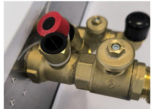
Safety valve PV-UT (see the hydraulic diagram of the internal connection) G 1/2" M x 3/4" F - supplied separately, attached to the T-piece intended for its installation - see the pic.
