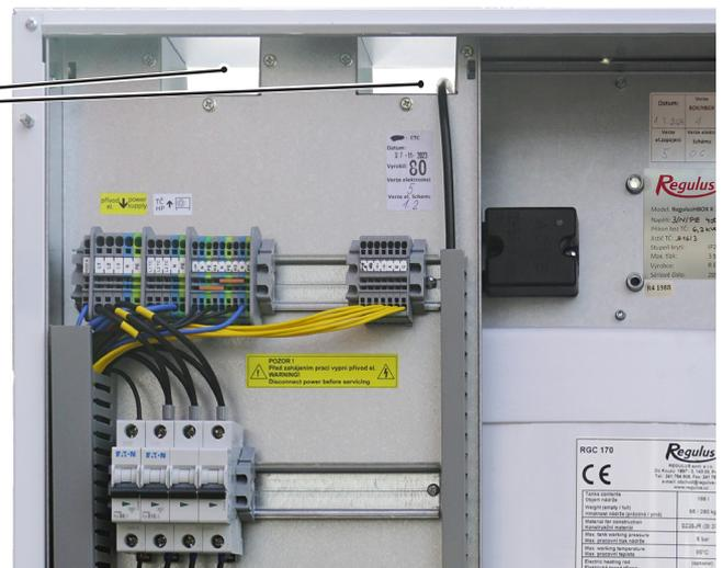
After closing the wiring cover, it is necessary to connect the control unit connector before refitting the front cover.
